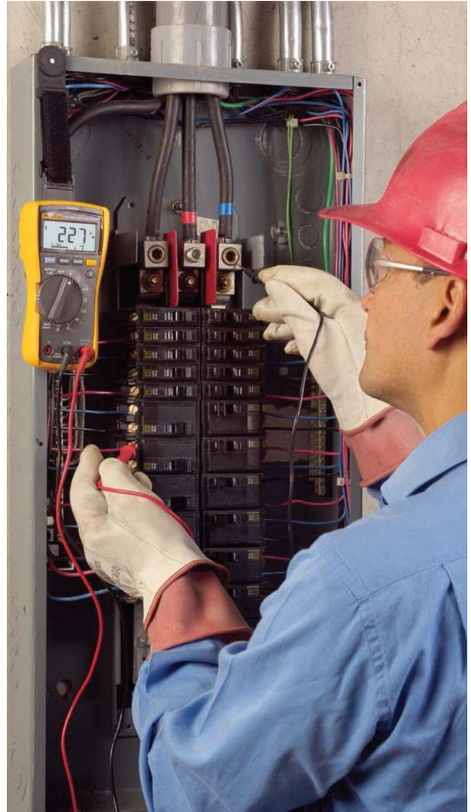
Low Z tools should only be used for testing power circuits or other circuits where low impedance will not negatively impact or alter circuit performance.
