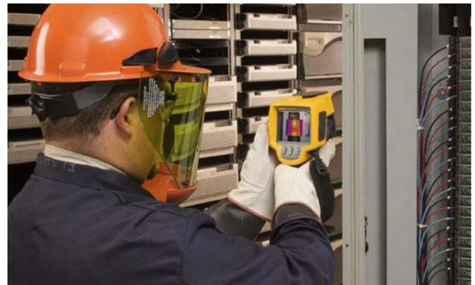
**Abnormally hot electrical connections are not only a potential early warning of failure and a safety hazard, they're also consuming excess energy.**
