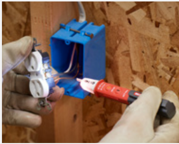
Test wires for AC voltage
